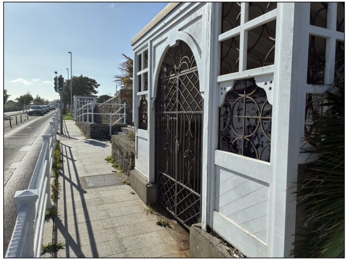
Two of the three Shelters by the East Pier
