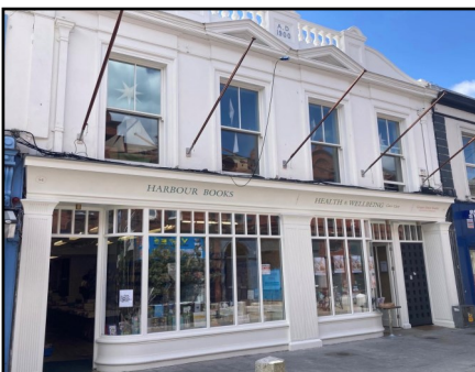
Before and After images of the refurbished shop fronts on
