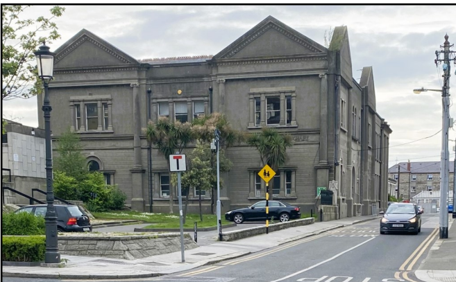
The Old Senior College Dún Laoghaire building which is being refurbished
